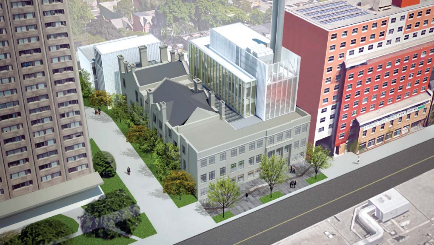
Exterior of the Centre for Urban Innovation
