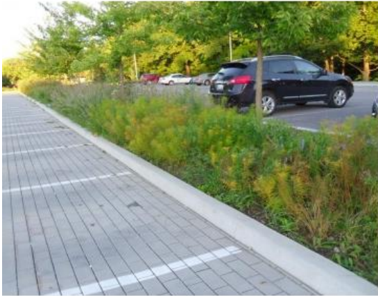
parking lot bioretention sharing underground reservoir with adjacent permeable paving, Edwards gardens, Toronto
