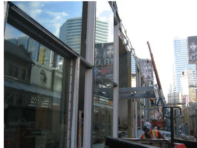
Retail glazing installation in progress
