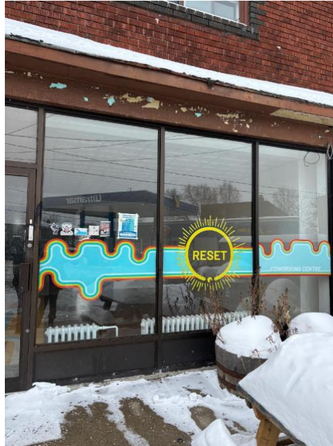
Figure 5: Image of a co-working space that is now vacant
