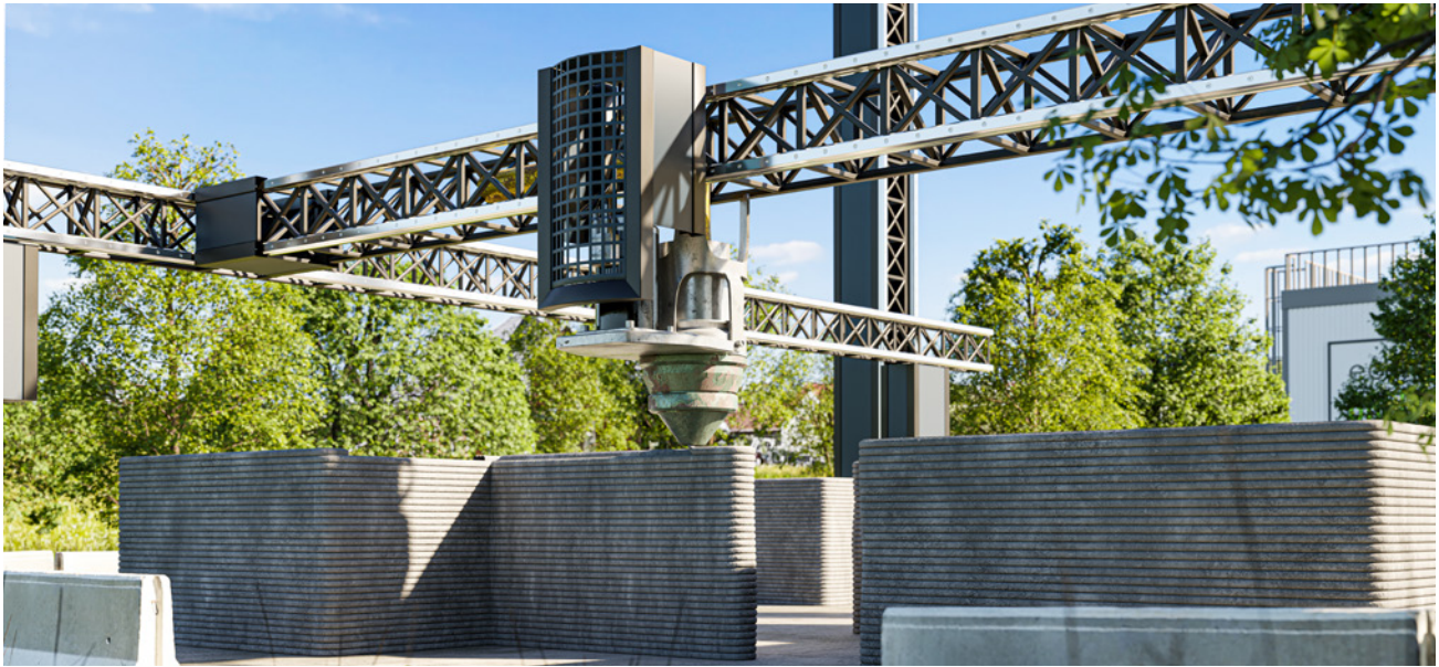
3D Printing a building with concrete.
