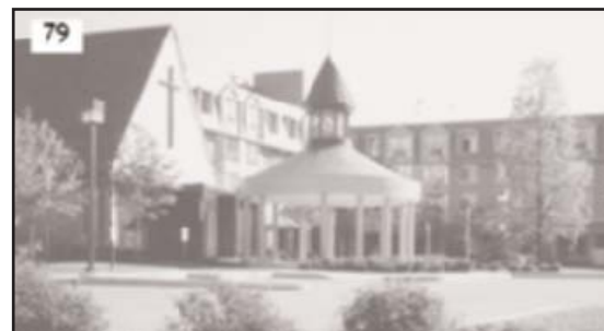
Front view of Humbervale Place
