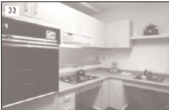
The same kitchen after removal of lower cupboards to enable users to work from a sitting position.
