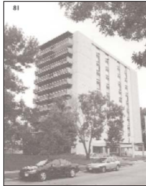
A view of ArlingtonHaus from the street
