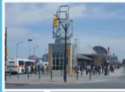
Transit Terminal Expansion
