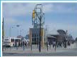
Transit Terminal Expansion
